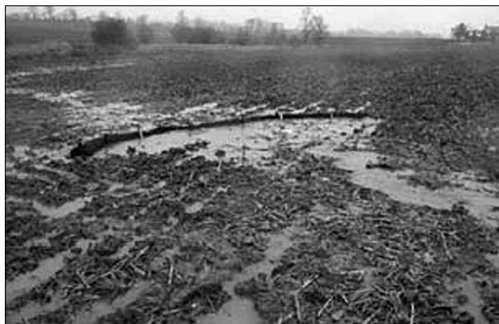
Figure 2. Filter sock accumulating water across a zone of concentrated flow during a rain in December, 2011
